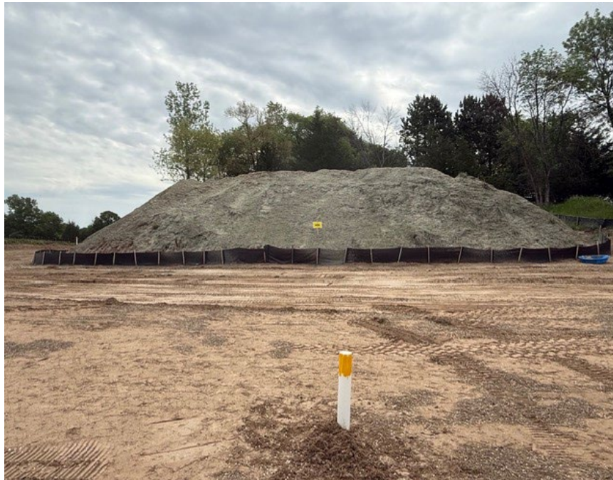
Facing east near MP 1.0, topsoil stockpile stabilized with hydroseed
