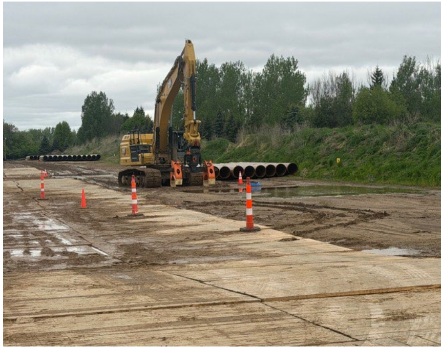
Facing west near MP 3.05, InterCon stringing new bore pipe
