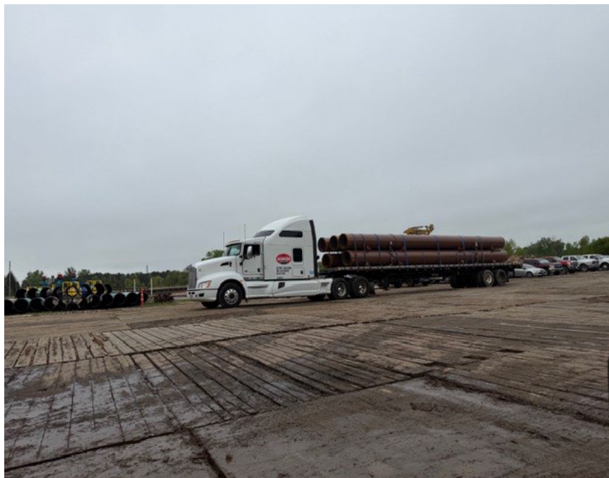
Facing south near MP 3.42, InterCon delivering new bore pipe
