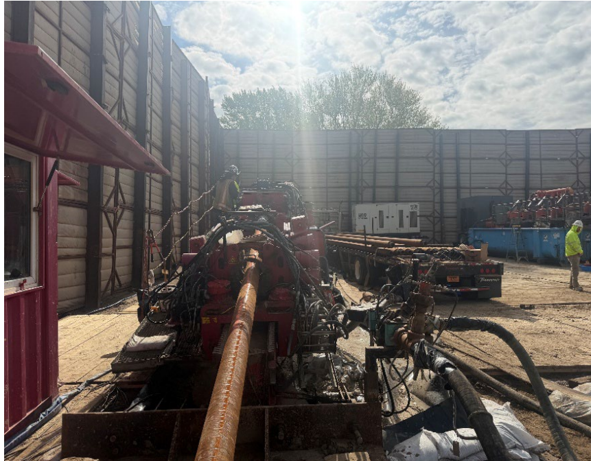
Facing east near MP 2.4, commencing the pilot hole on HDD P4-5
